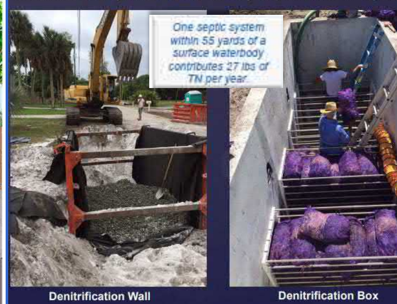
Micco/Little Hollywood Water Quality Improvement Project
